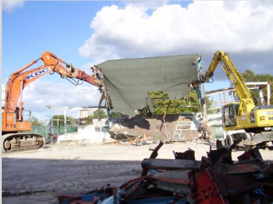
Use of plant to bring down building frame
