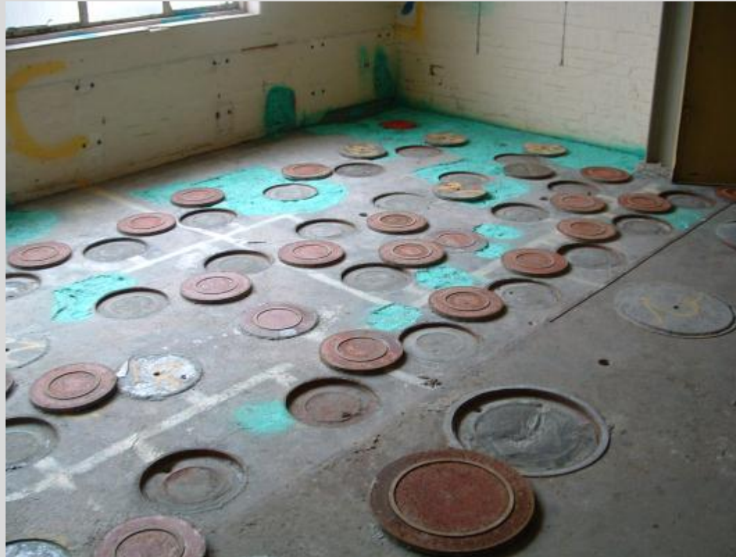
RSRL immobilisation of contaminated storage tubes
