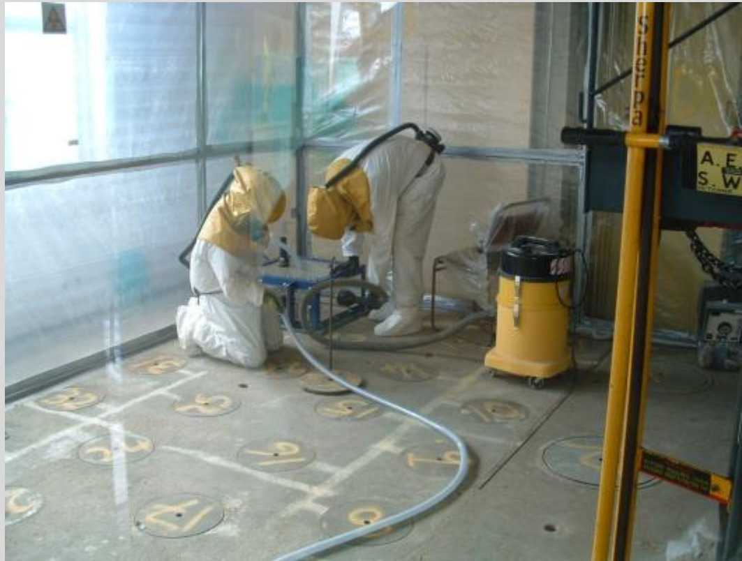
RSRL immobilisation of contaminated storage tubes
