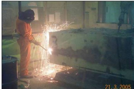
De-cladding cave station blocks using a Petrogen Oxy-gasoline torch (WBS_4.15.2-4.2.8)
